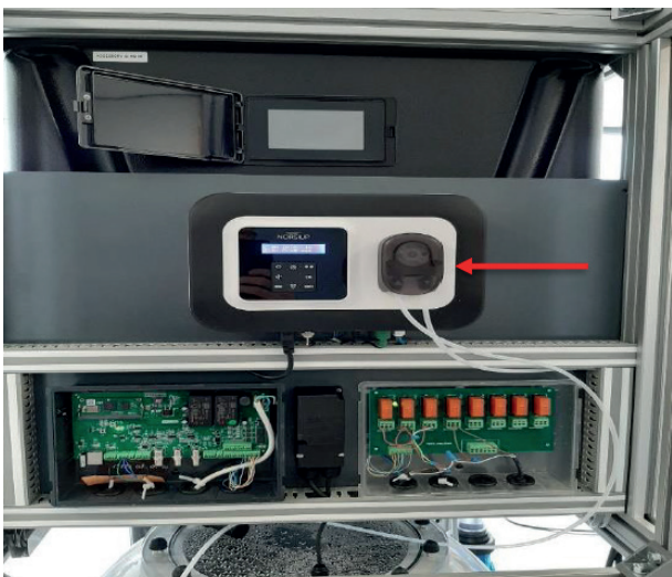
Fig. 13: Shows the Salt Chlorinator
